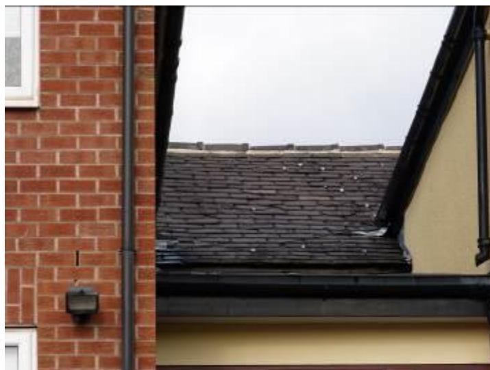
Cracked and slipped slates to rear roof slope, visible between modern extensions
