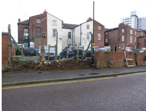
Damaged rear wall behind Birkdale and Chester Terraces
