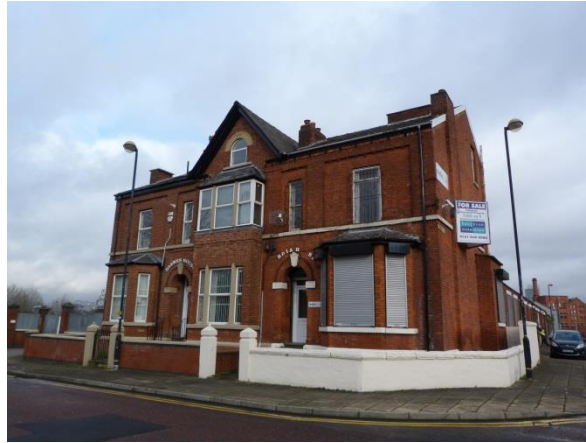
Nos 4 and 6 Darwen Street
