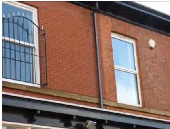
Building join where the Flemish bond brickwork of the original 19 th -century terrace meets a late 20 th -century stretcher bond addition
