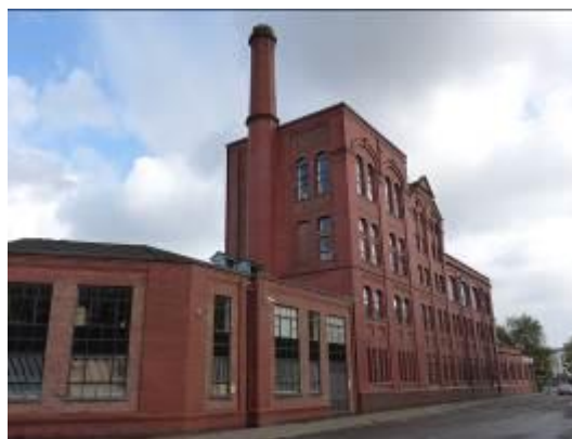
The modern extension on west side of the Empress Building with notably larger windows and mismatching stringcourses.
