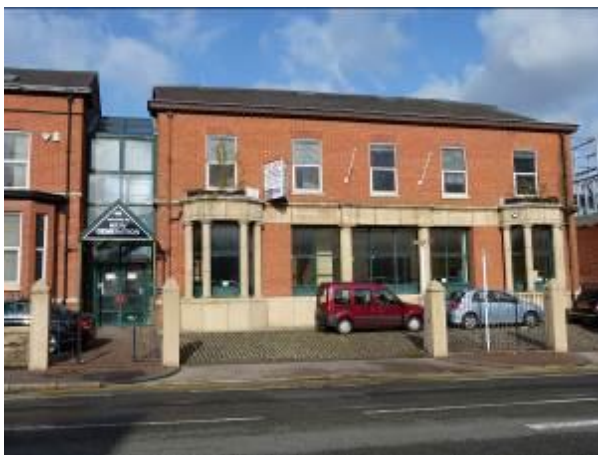
The modern shop front on Chester Road
