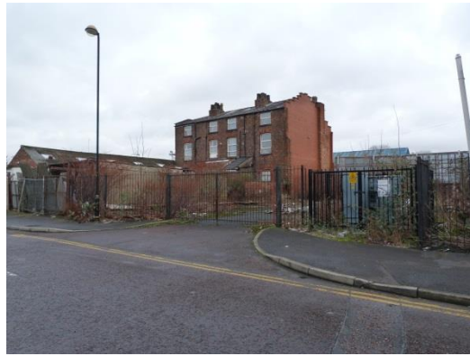
Rear of Cornbrook Terrace and adjoining vacant plot
